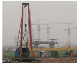
Figure 3 GPS-10 Bored Pile Drill
