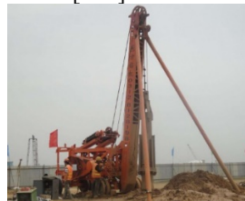
Figure 2 CZ-8 Wire Rope Percussion Drill
